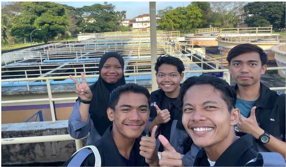
An Overview of the Tanks
