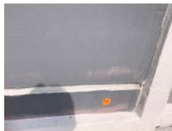
P66- Uneven paint surface on the wall
