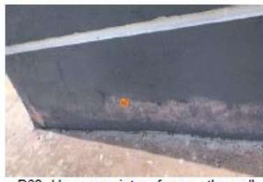
P63- Uneven paint surface on the wall
